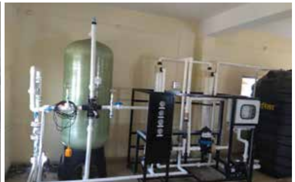
RO plant of 5000 lits/hr capacity set up near the lake at Ausa under DST project
