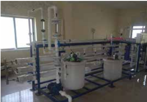
RO plant of 5000 lits/hr capacity set up near the lake at Ausa under DST project
